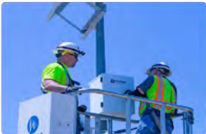
LIGHTING AND SIGNAGE
