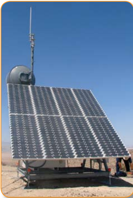
This 1200 watt SunWize Power Station located in a remote location, powers telemetry equipment
